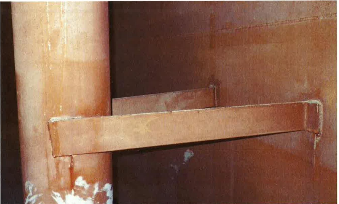
66. Inlet pipe bracket.
