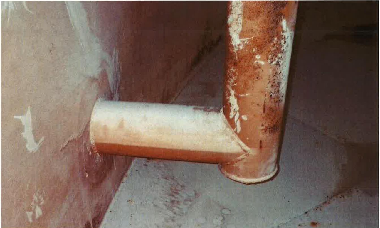
64. Overflow pipe penetration through shell.
