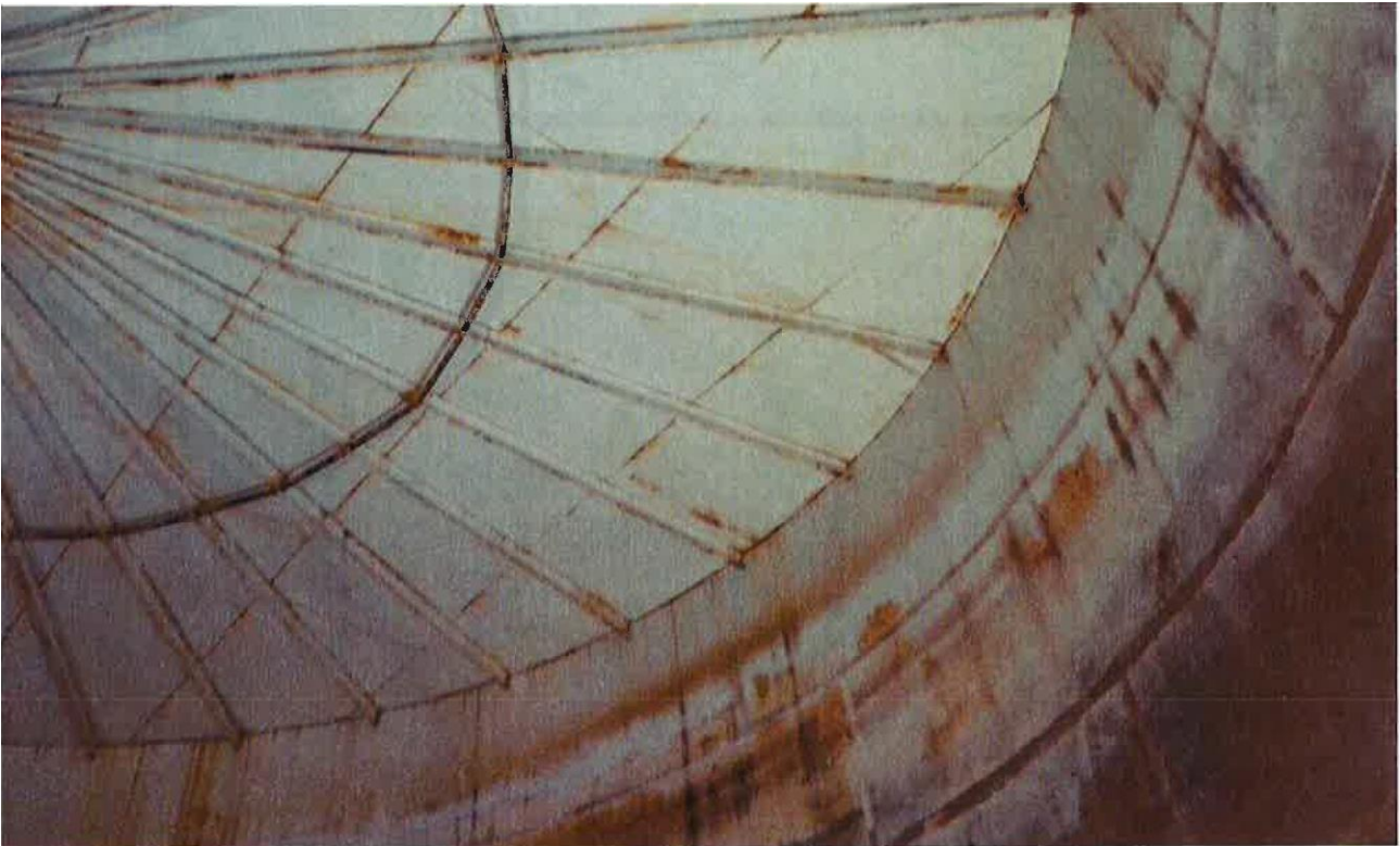
50. Roof and roof support structure.
