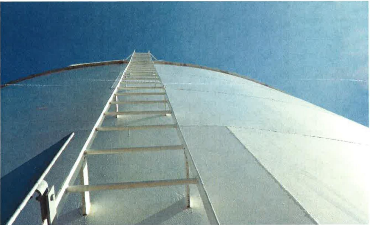
35. Exterior shell ladder.
