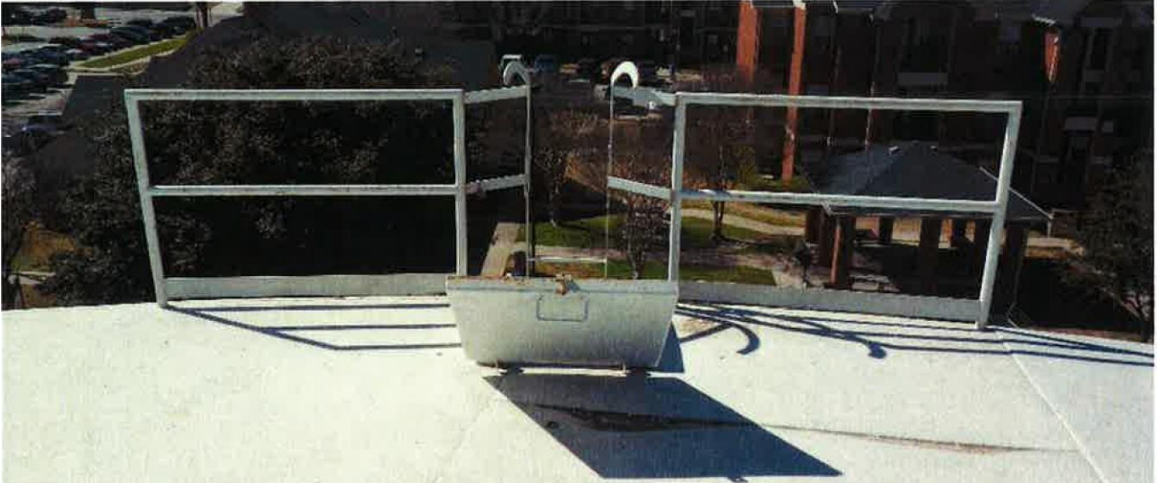
38. Roof manhole, roof safety railing, and access opening.
