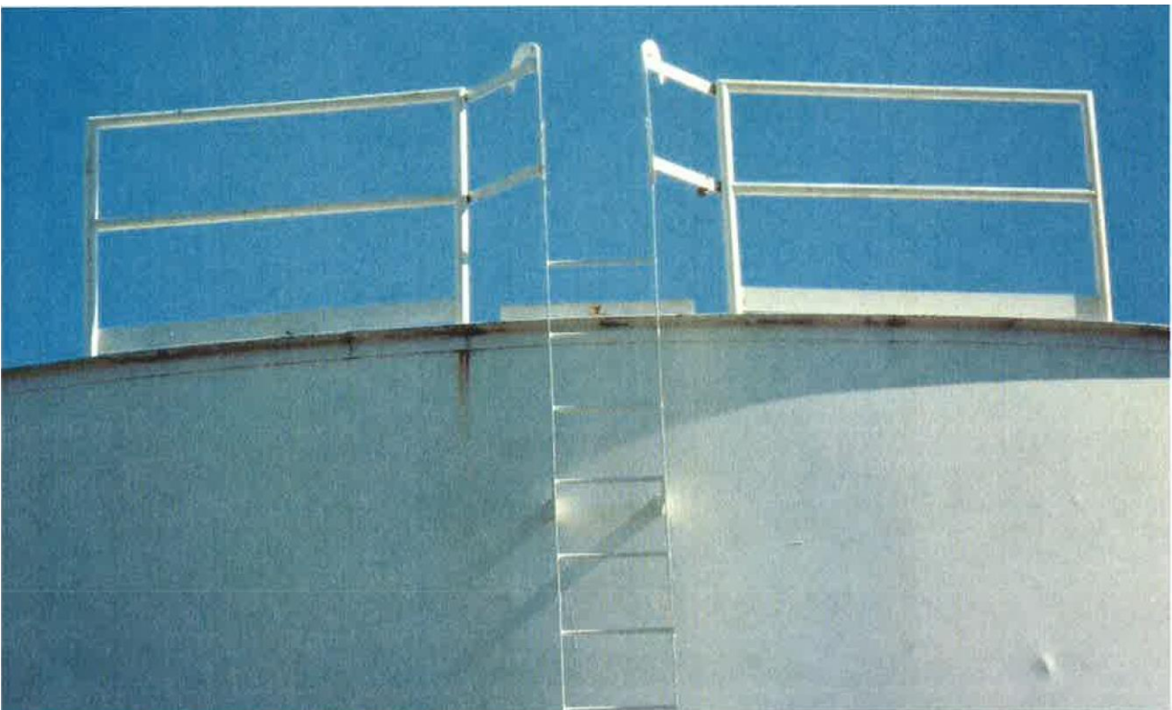
36. Exterior shell ladder, roof safety railing, and access opening.
