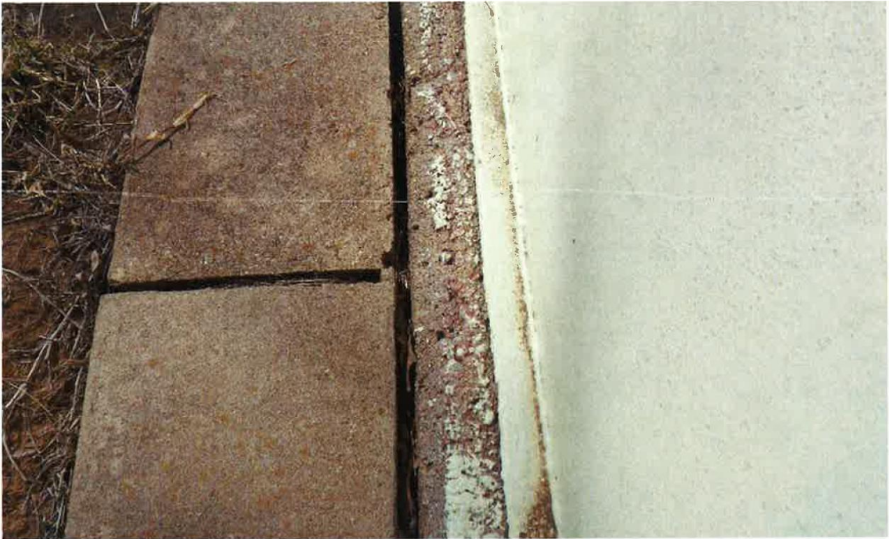
13. Bottom plate and foundation.
