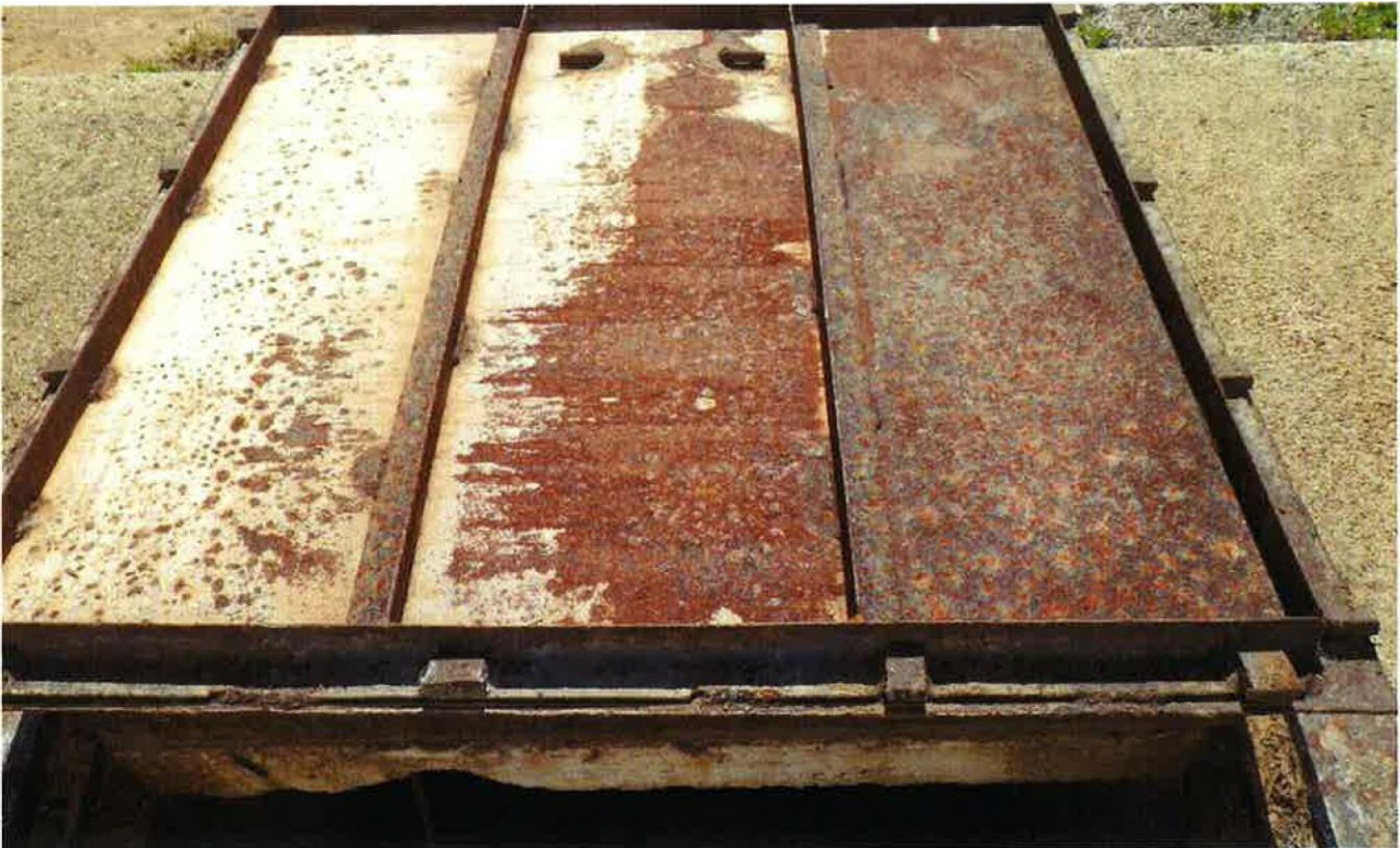
6 . Valve vault cover.
