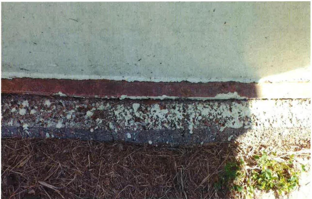
10. Bottom plate and foundation.
