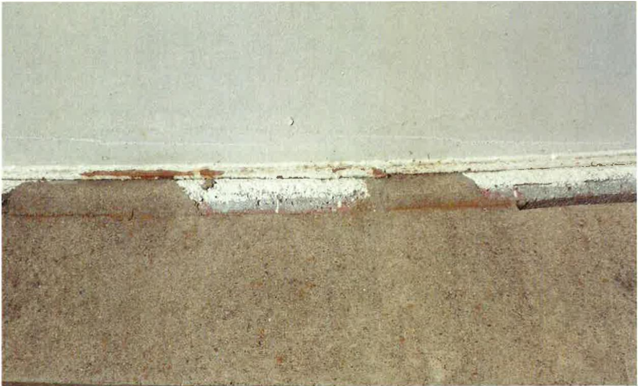
15. Bottom plate and foundation. Note coating on repaired foundation.
