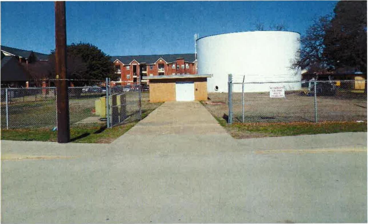
3. Entrance to site. Note sign on fence.
