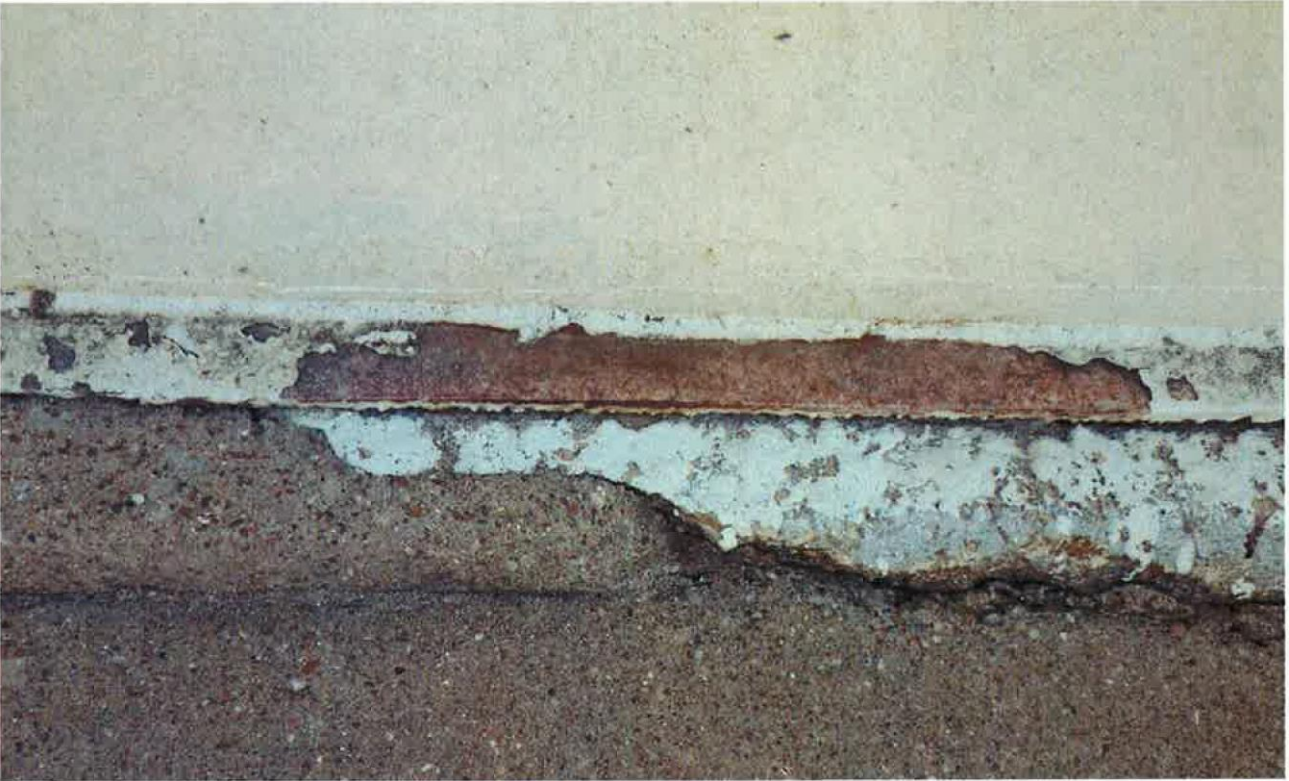
11. Bottom plate and foundation.
