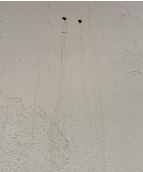
Water Damage to Entry Ceiling
