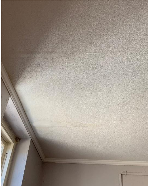
Water Seeping Through Mortar During Heavy Rain
