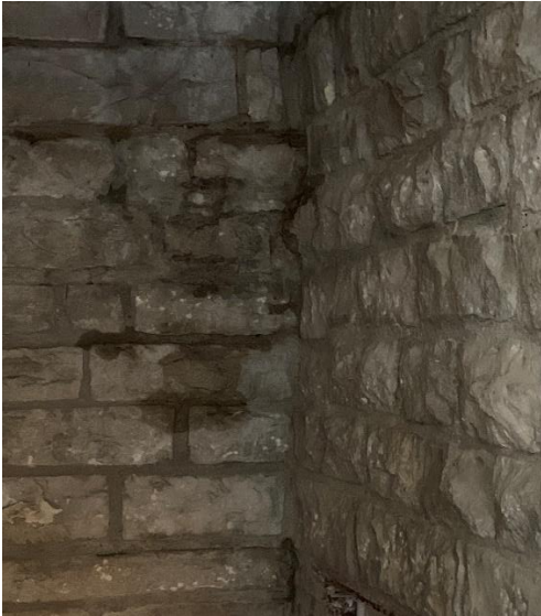
Water Seeping Through Mortar During Heavy Rain
