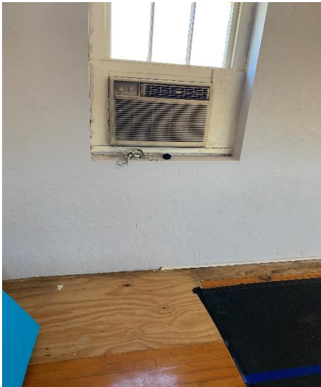
Water Damage to Wood Floor Along Walls
